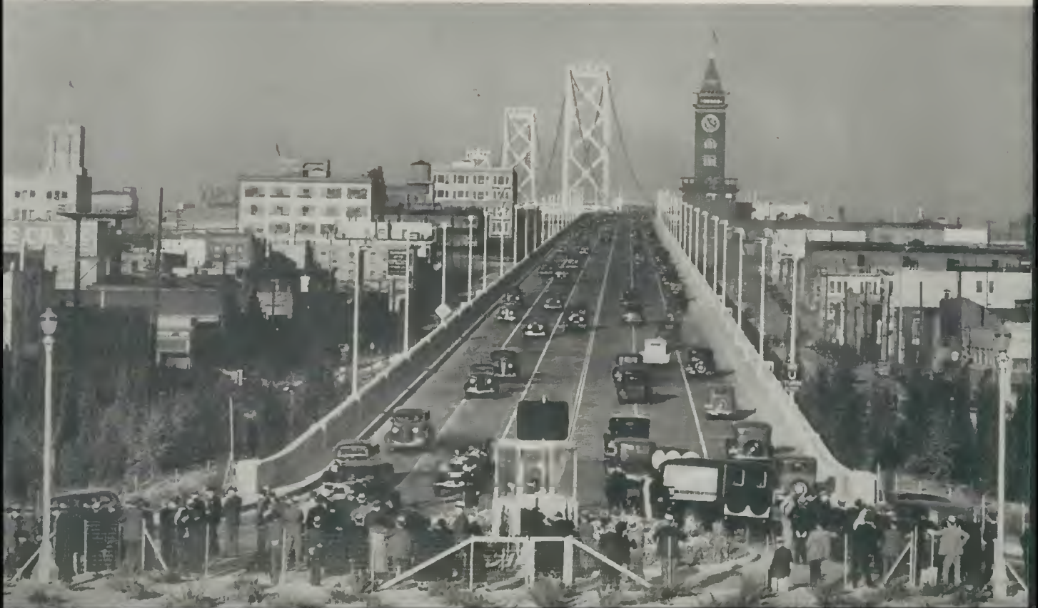
LOOKING EAST ON THE BRIDGE FROM FIFTH STREET PLAZA, SAN FRANCISCO
