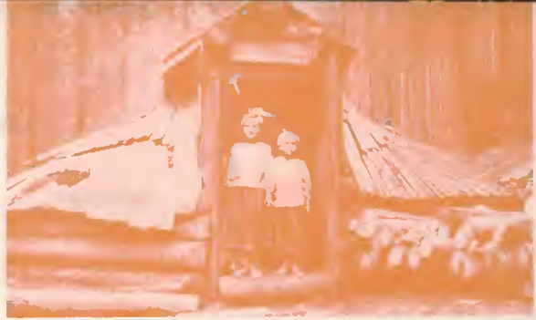
The forest hut of a Hucul woodsman. These koli-bri are circular with a hole in the center of the sloping roof. Food, mostly cornmeal bread and salt pork, is cooked over a simple fire directly under the opening in the roof. The members of the family sleep on pine branches, feet to the fire.
