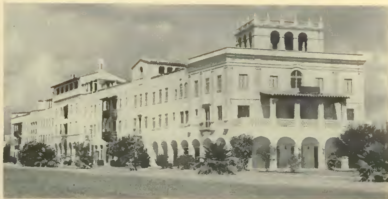
Administration Building and Women's Residence Hall of the University of Miami.
