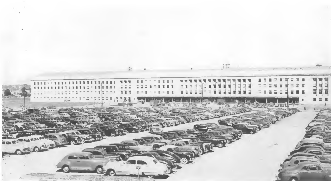
View of south parking lot showing loading platform to maintenance area of building
