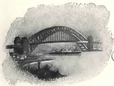
Sydney Harbor Bridge
