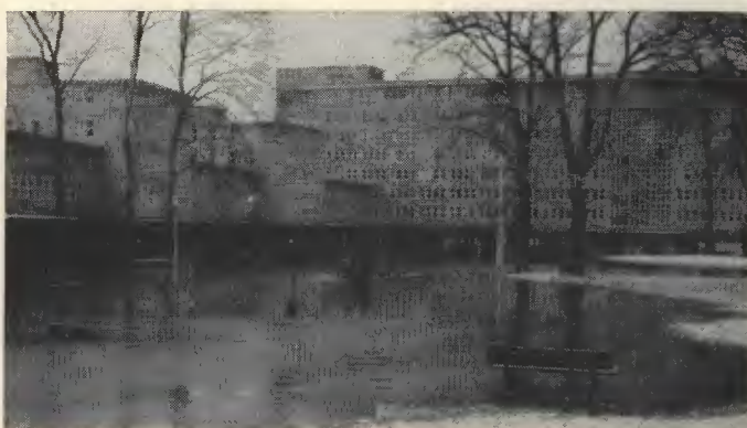
The flooding of the grounds of the Chancery in Bonn-Bad Godesburg during the recent floods.
